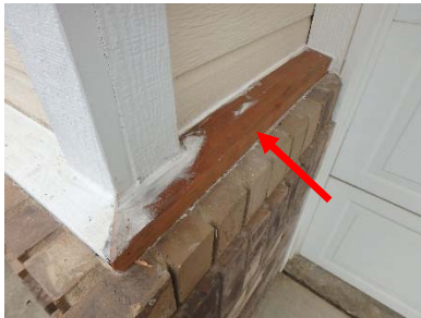
Trim at Garage
