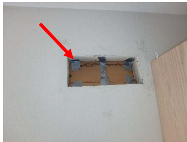
Right Side Wall in Garage
