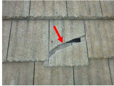
Damaged Tile
