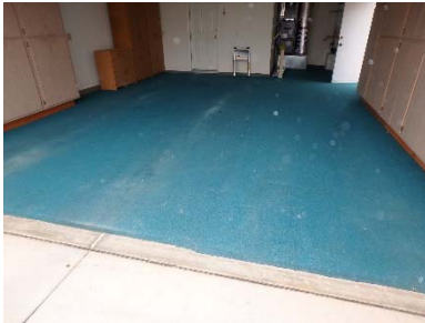
Carpeting on Garage Floor
