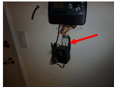
Right Side Garage Wall
